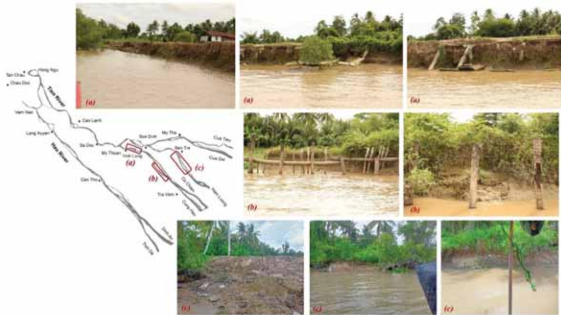
Figure 4. The riverbank erosion locations along the VMD River.
